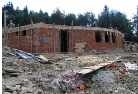
Litmanova enclosed building under construction
