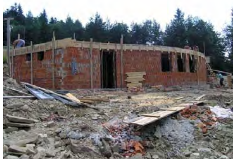
Litmanova enclosed building under construction
