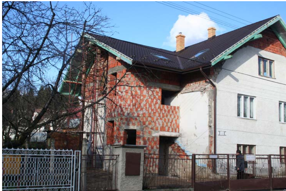
New roof and new stairs
