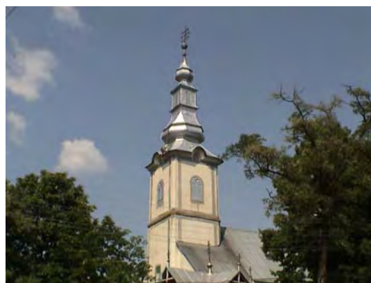
The completed job! Thank you for supporting the work of the Mission Society.
