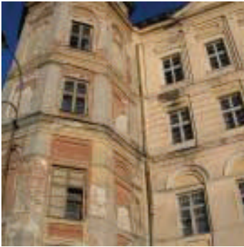
One of the towers before restoration work began
